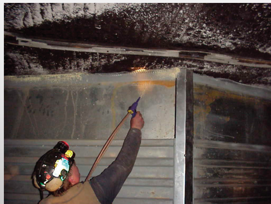
SEAL METAL STOPPINGS
